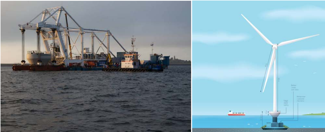
Figure 3.4. Left: Placement of foundation on the seabed by means of a large floating crane. Right: schematic drawing of turbine mounted on the foundation, which is placed on top of the gravel bed and held in place by ballast rocks. The foundation is protected from scour on the sides. The inverted cone at the top helps to protect the foundation against ice in winter. Photo and graphics: Sund&Bælt A/S.
