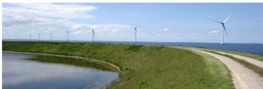
Figure 3.3. Turbines seen from north-eastern tip of Sprogø Photo: Sund&Bælt A/S.
